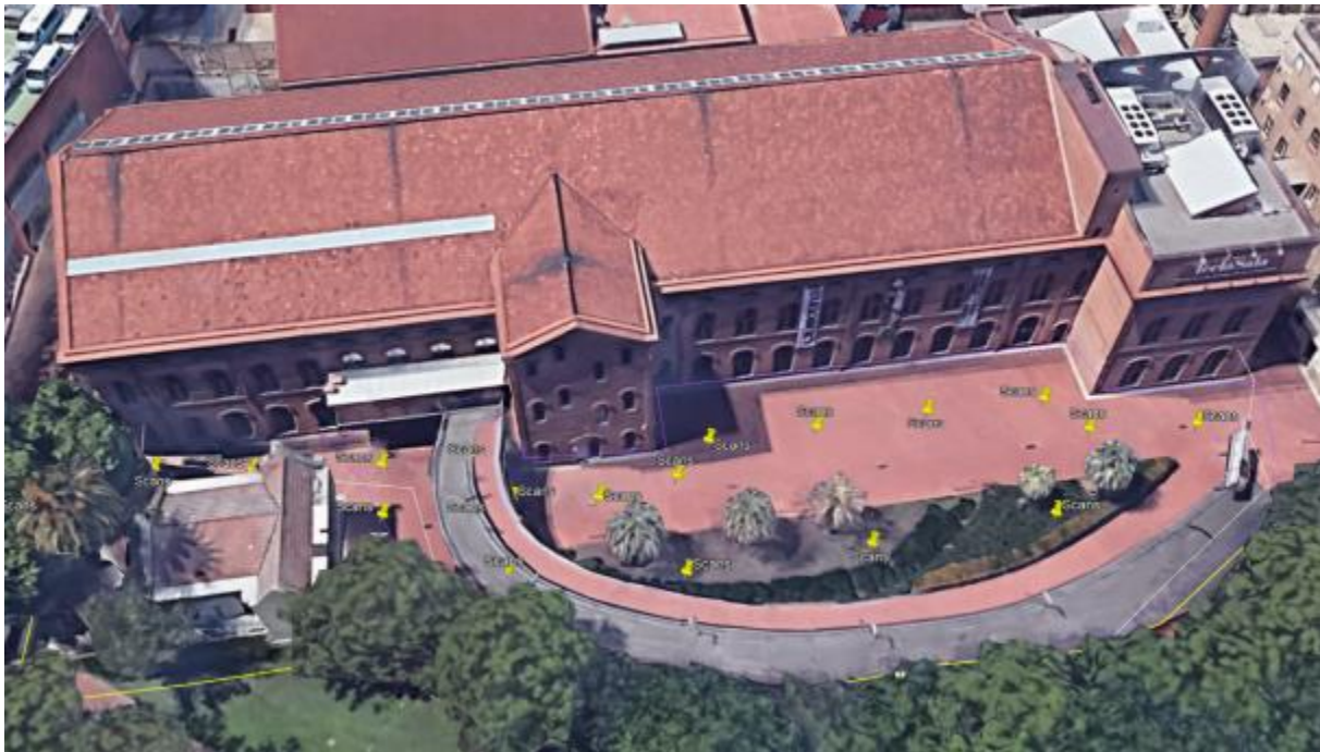
Figure 54. Planning of scan stations for the 3D scanning survey by means of a terrestrial laser scanner
